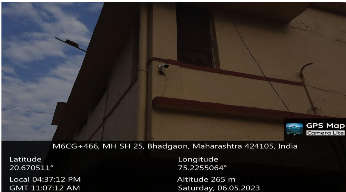
CCTV Camera in Old Campus
